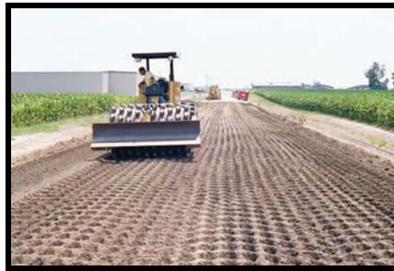
(Fig 2: Fly Ash used in Soil Improvement)
